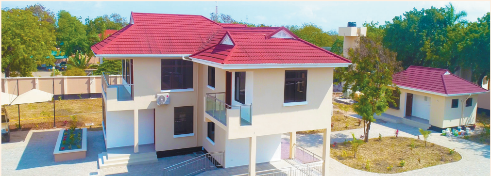
Residential House for Government Officials
